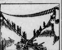
A recent cloudburst near Telluride Col., swept all the supporting work of these tracks away, leaving the rails and ties suspended over a deep gulch. Nearly 200 feet of track was thus left suspended, and only the timely discovery of the washout prevented a Denver & Rio Grande railroad train from running into the gulch.-Popular Mechanics.
