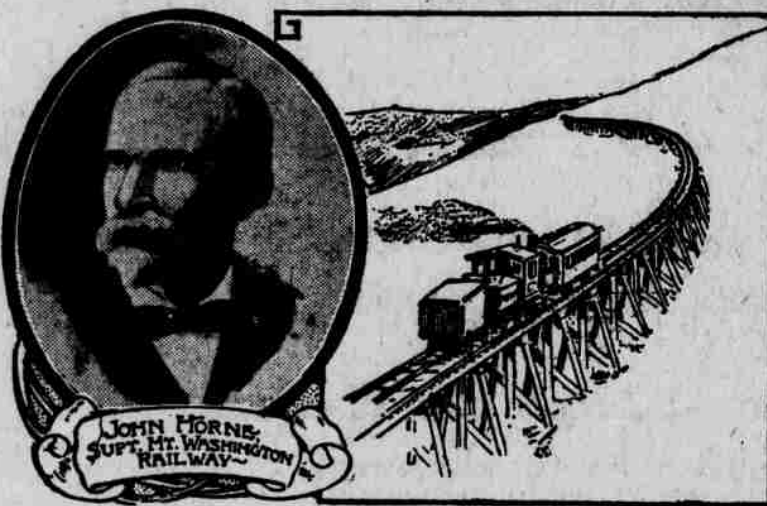
Line from the Base to the Summit of Mount Washington Is Really a Fine Piece of Engineering—Superintendent Tells of the Work Done on One of the Regular Trips—Is Strikingly Original in Construction.
