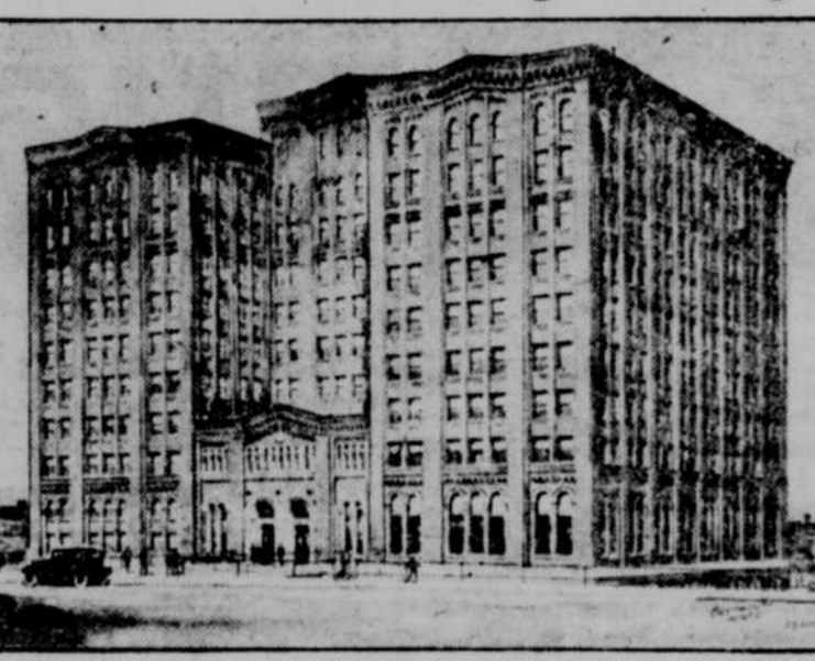
This new building now under construction at South Omaha will be one of the largest and best equipped livestock administration buildings in the world.
