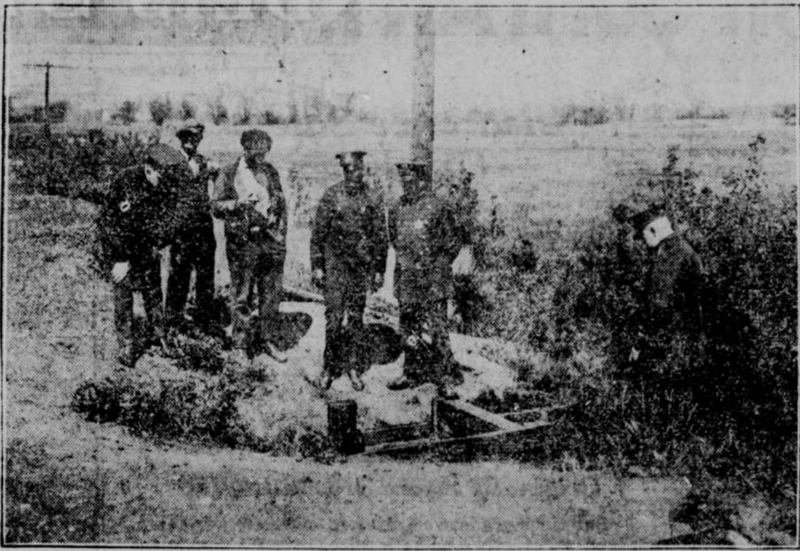
Beneath this culvert at One Hundred Twenty-first street and the Pennsylvania tracks, Chicago, was found the body of Robert Franks, 13-year-old son of Jacob Franks, millionaire. The kidnapers had demanded $10,000 ransom.
