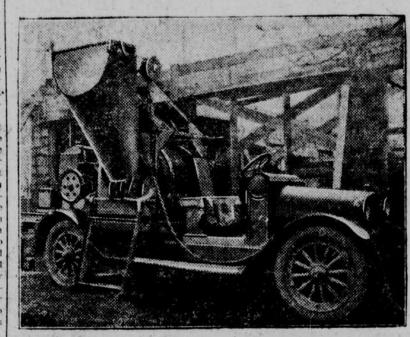
of a mounted mixing machine. Leavens mounted a 10-foot mixer, average machine used by contractors he can eliminate a lot of handling Car company.
