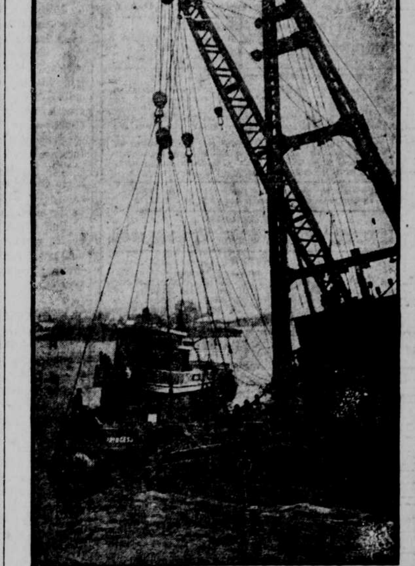
Hosts created and salvage barges tipped dangerously close to water's edge as tugboat Princess, which sank off Hoboken, N. J., was lifted from water. In engine room of tug was found the body of engineer, who had been trapped when the Princess went down.
