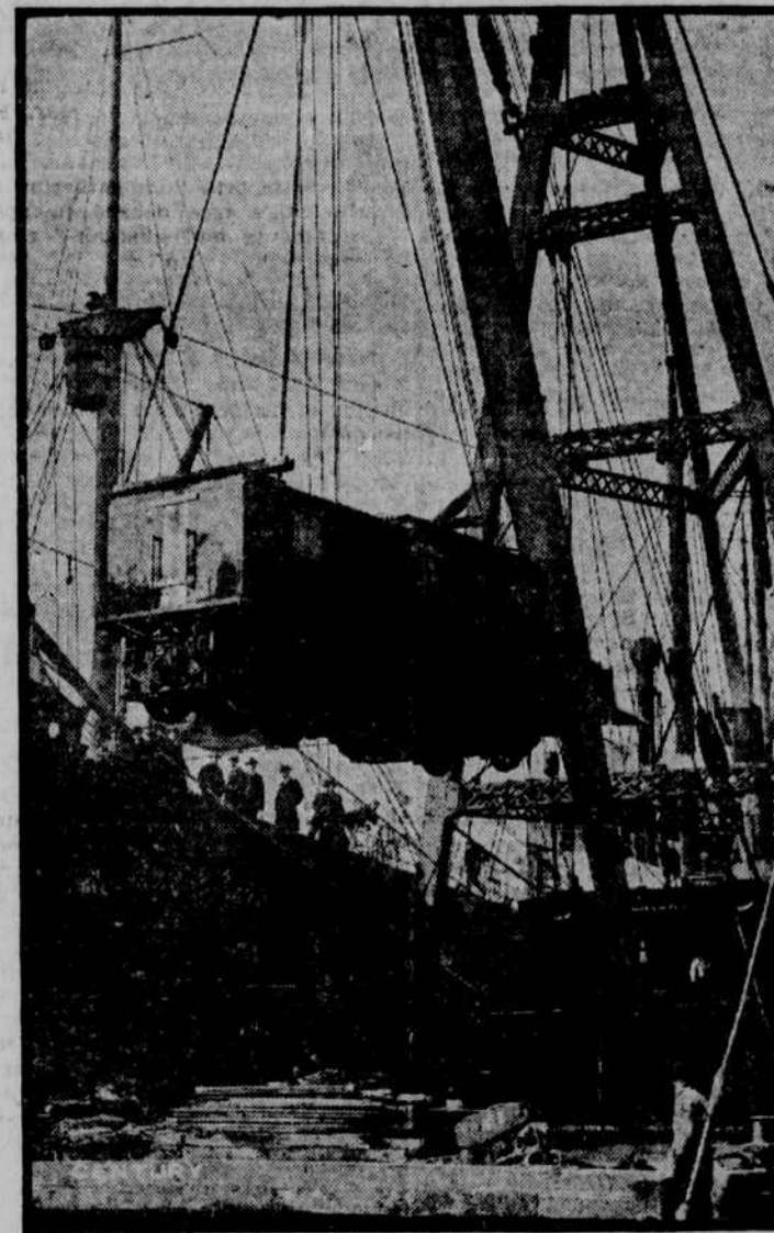
Photo shows one of two 70-ton electric locomotives which were lifted into the hold of the French steamer Ontario by giant hoists at pier in North River, New York, for use in Europe. Usually engines are shipped un-assembled.
