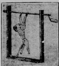
holes. Make your handle of a piece of wire bent into end of spool and fasten to one end of the cross pole.
