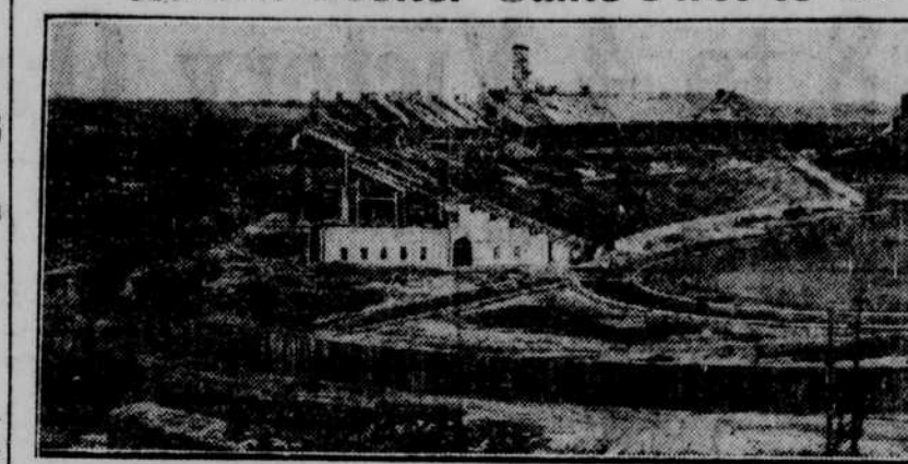
Here is the Nebraska stadium as it looks today. All day Friday workmen hurried to put the giant structure into shape for the much-talked-of game. The great structure is capable of seating 30,000 persons at all times and 47,000 persons when the temporary seats are installed. It is built of concrete and steel and has a circumference, outside the running track, of 2,100 feet. The farthest seats are 215 feet from the sidelines. On Homecoming day, October 20, the structure will be dedicated. Thousands of alumni are expected to return to their Alma Mater for the services. No definite date has been set for the completion of the stadium. The committee in charge declares this impossible at this time.
