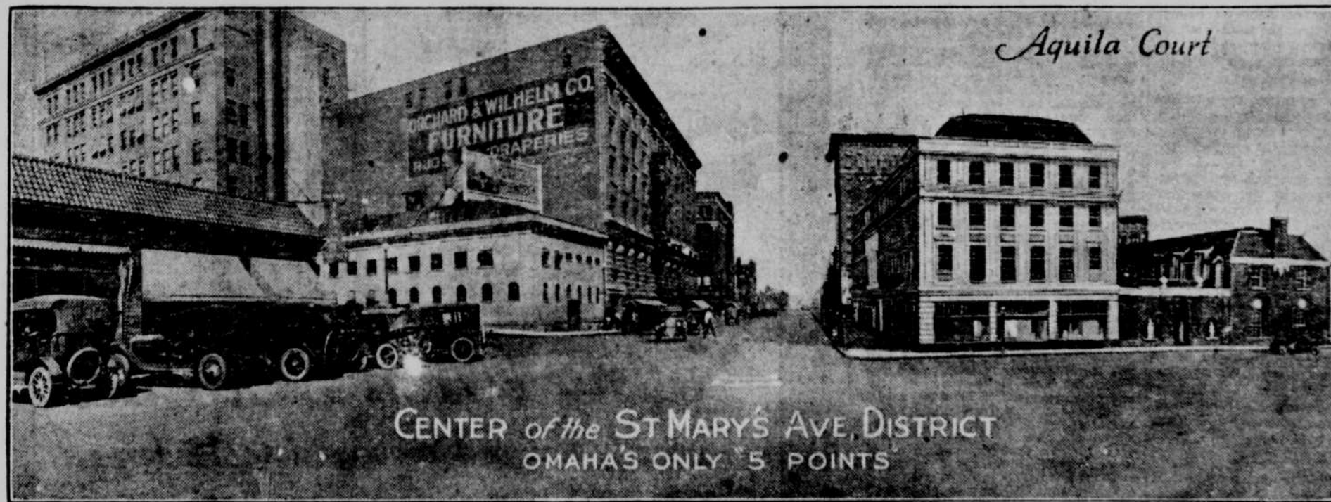
Showing where the distinctive and beautiful Aquila Court Buildings will be located. (Photograph of Aquila Court in exact perspective, though building not yet complete.)
