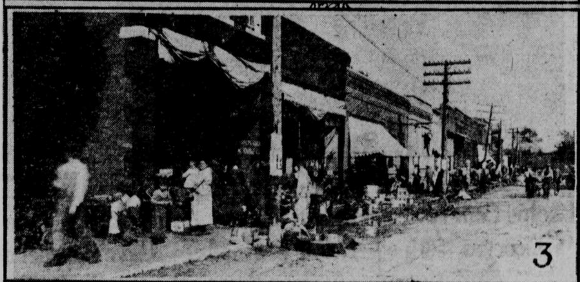
Work of reconstruction at Louisville, Neb., was under full steam Monday, following the ravages of Friday's storm, in which 12 lives were lost.
