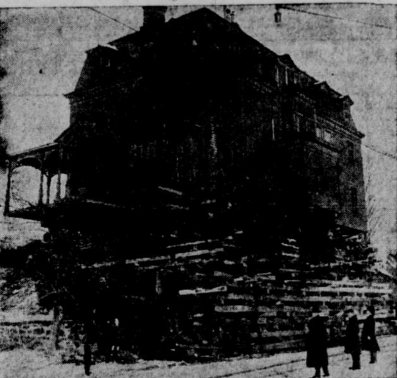
An old mansion which was built in the revolutionary days, was moved across the street in Brooklyn, N. Y., and had to be raised 25 feet to avoid blocking traffic.
