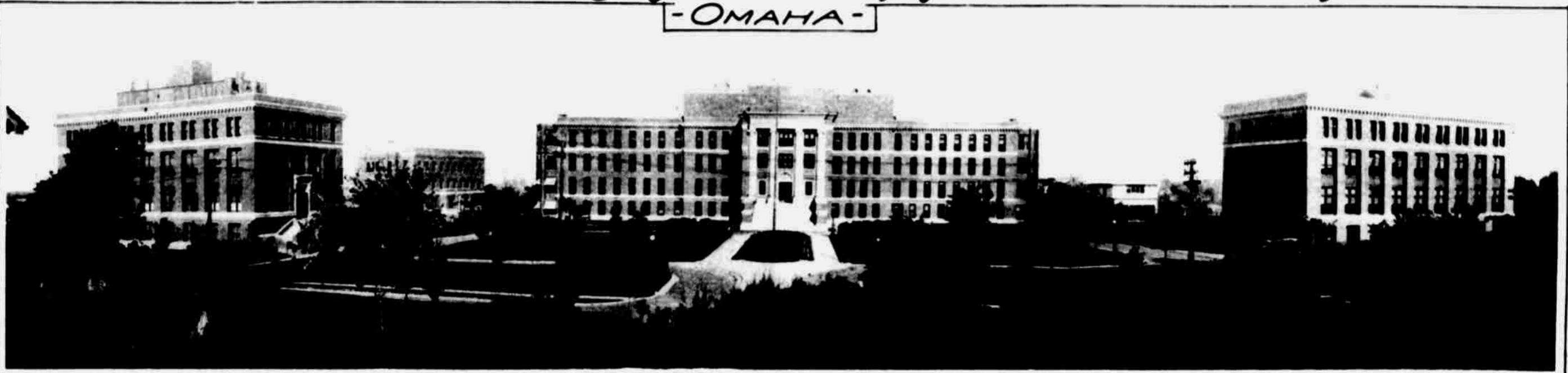
South Laboratory Building
