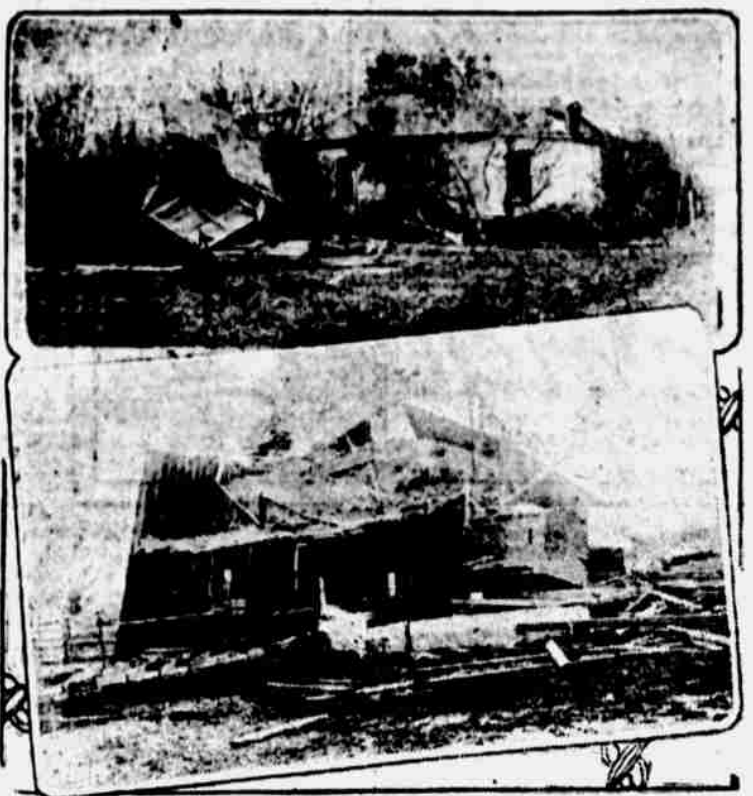
Monday night's tornado played pranks when it reached the farm of C. H. Warner, three miles south of York, Neb. After wrecking the barn, the storm piled debris around the yard and uprooted trees, but scarcely touched the house.
