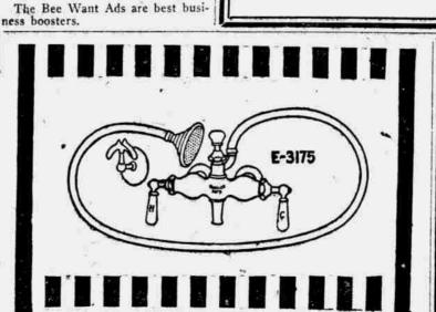
The newest plumbing fitting — the MUELLER Tub-Shower Faucet-gives you a shower bath or a tub bath at your option -simply raise or lower the center knob and you get hot, cold or tempered water through spout or spray-the hose is permanently attached-insist on this faucet for your new tub or have it installed on your old tub.
