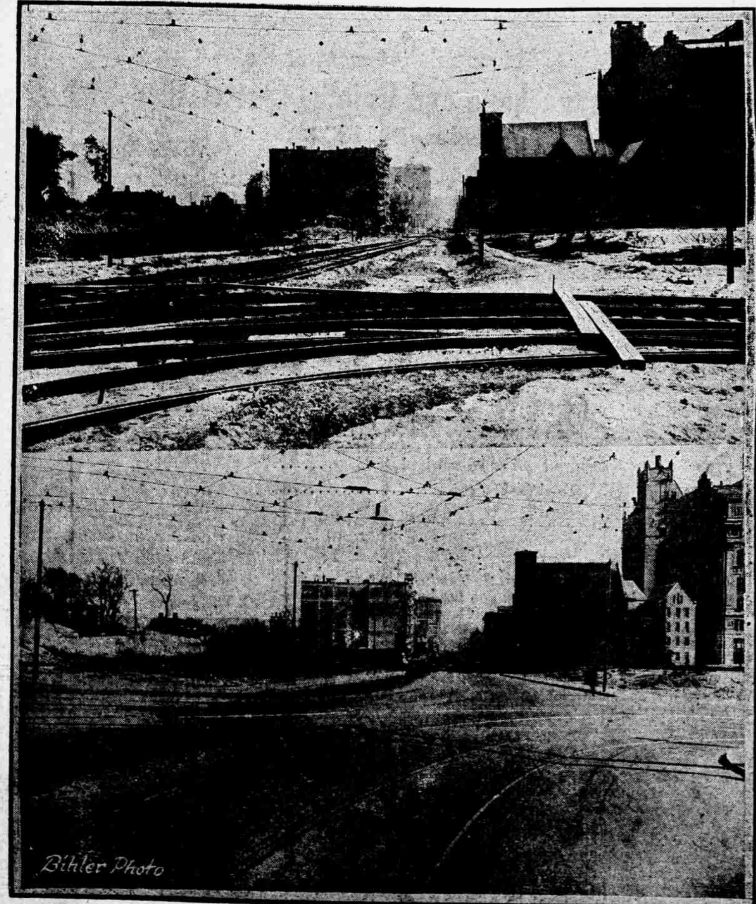
Twentieth and Dodge streets before and after. What an improvement is made by good paving is convincingly shown in the above photographs. This paving was laid in 38 days by the American Paving corporation. It cost $25,000 less than it would have cost a year ago. It is vitrified brick block, which the contractor explains means permanent paving in every respect. It is pointed out that brick laid on Dodge street west of the Poony farm 26 years ago is still standing up. The vitrified brick made now days is a much superior product to the brick made a quarter of a century ago, too.
