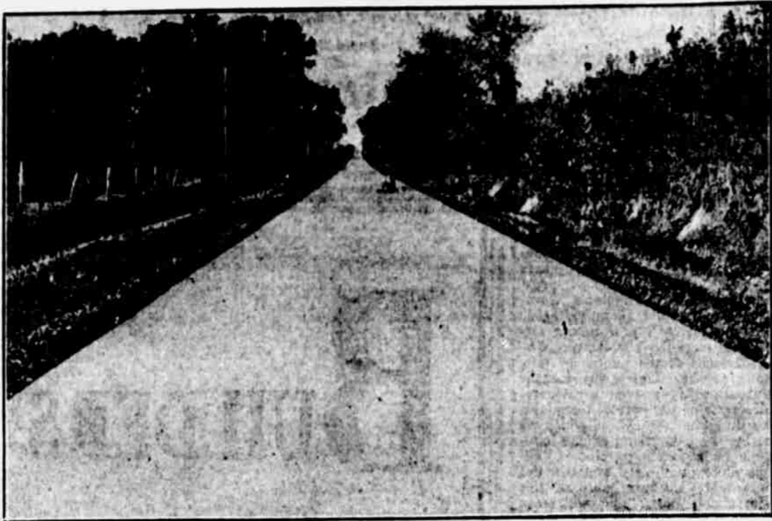
The road to Fort Calhoun north of Florence. This highway has been recently paved under the Douglas county appropriation.
