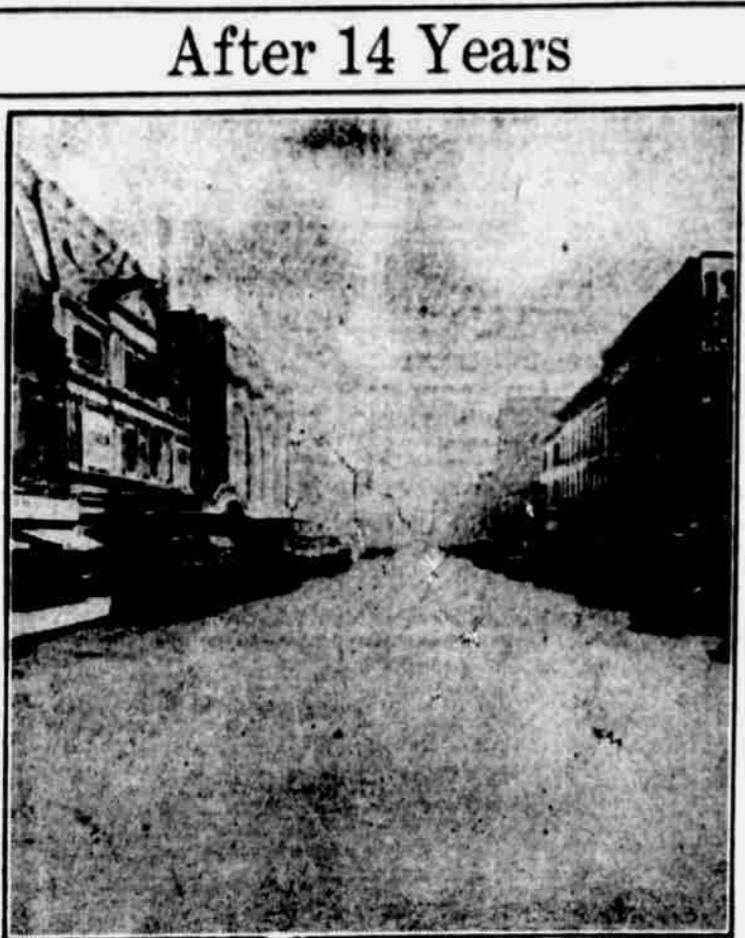
After 14 Years After 14 years the asphalt paving laid by Hugh Murphy on Douglas street east from Sixteenth street is still withstanding the battering of downtown travel. The paving is two inches of sheet asphalt laid on a 14-inch concrete base with an inch and a half of filler. It's almost as good as the day it was laid.
