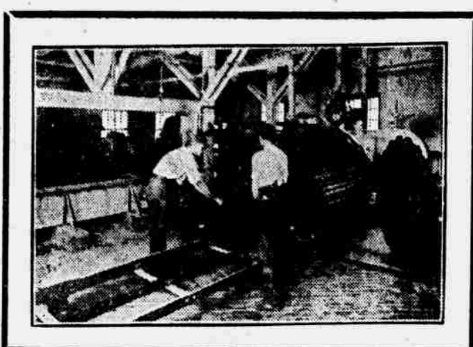
Another section of the tuberoom.
