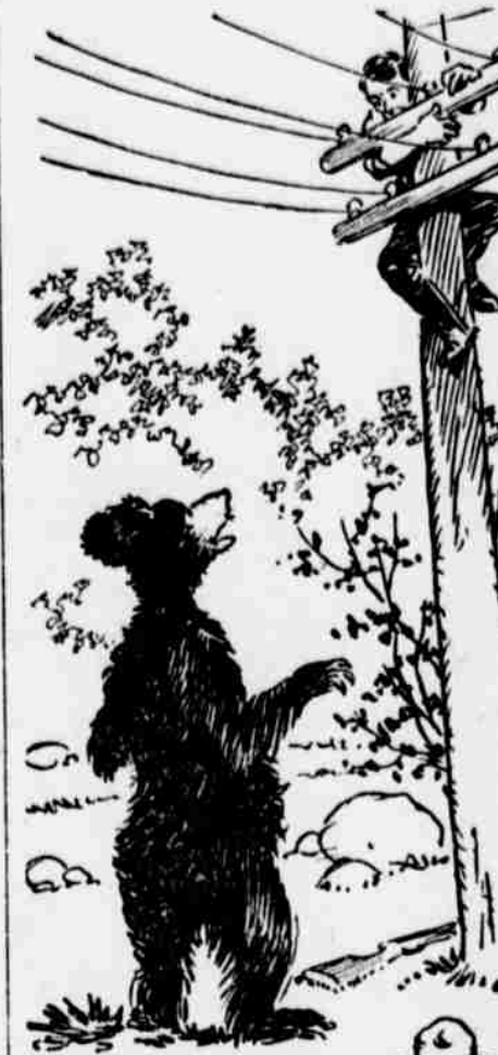
"Paraded Around That Pole for Two Mortal Hours."
