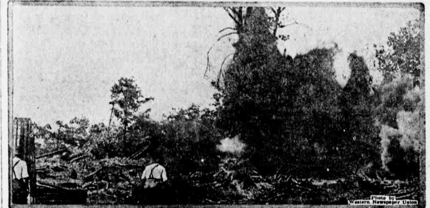
At Newark, N. J., a small army of men is busily engaged in clearing Heller field which, when completed, will be the first United States aerial mail landing field in the country. Our photograph shows the moment of detonation of a charge of dynamite beneath a mighty tree stump, which is torn from the grounds, roots and all.
