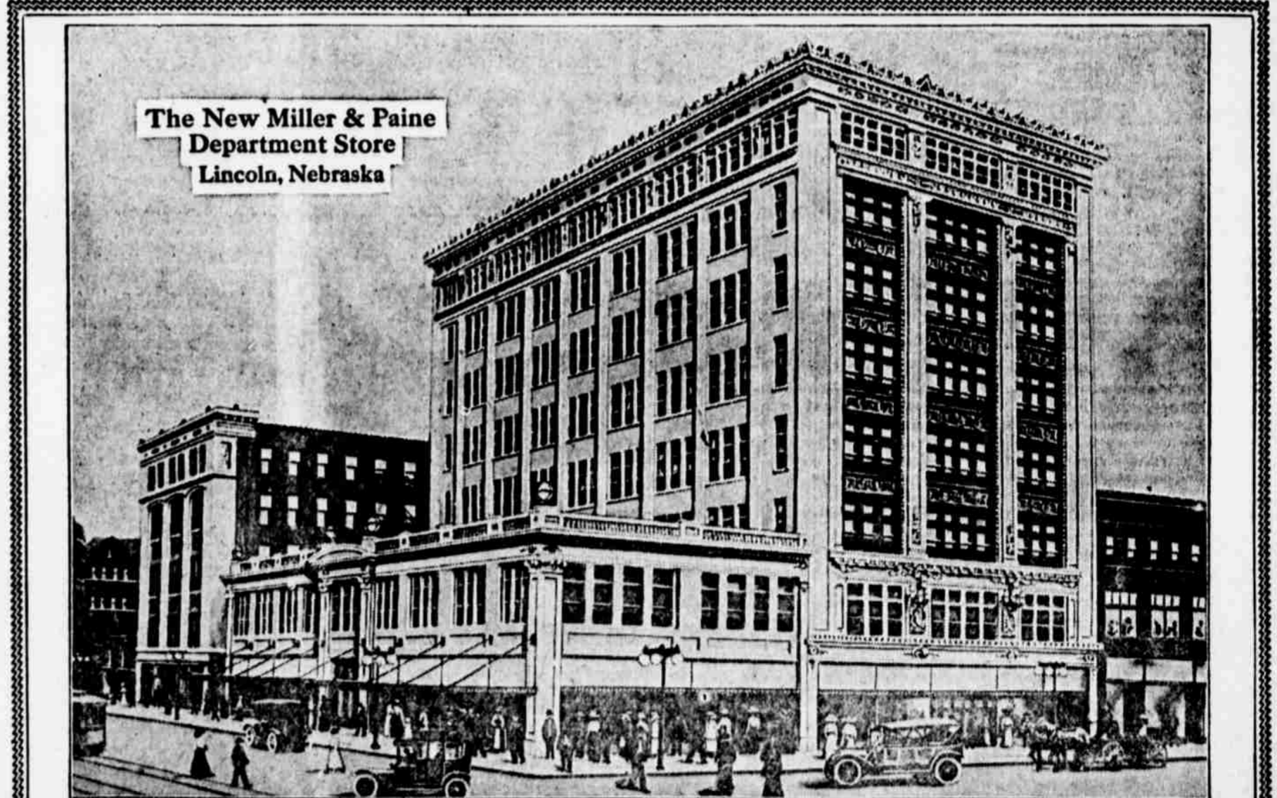
This modern fire-proof building occupied exclusively by Miller & Paine Department Store. Built of buff brick and ivory-colored terracotta, with green trimmings. Includes nine floors (3 1/2 acres of floor space.) Height to top of tower, 156 feet.
