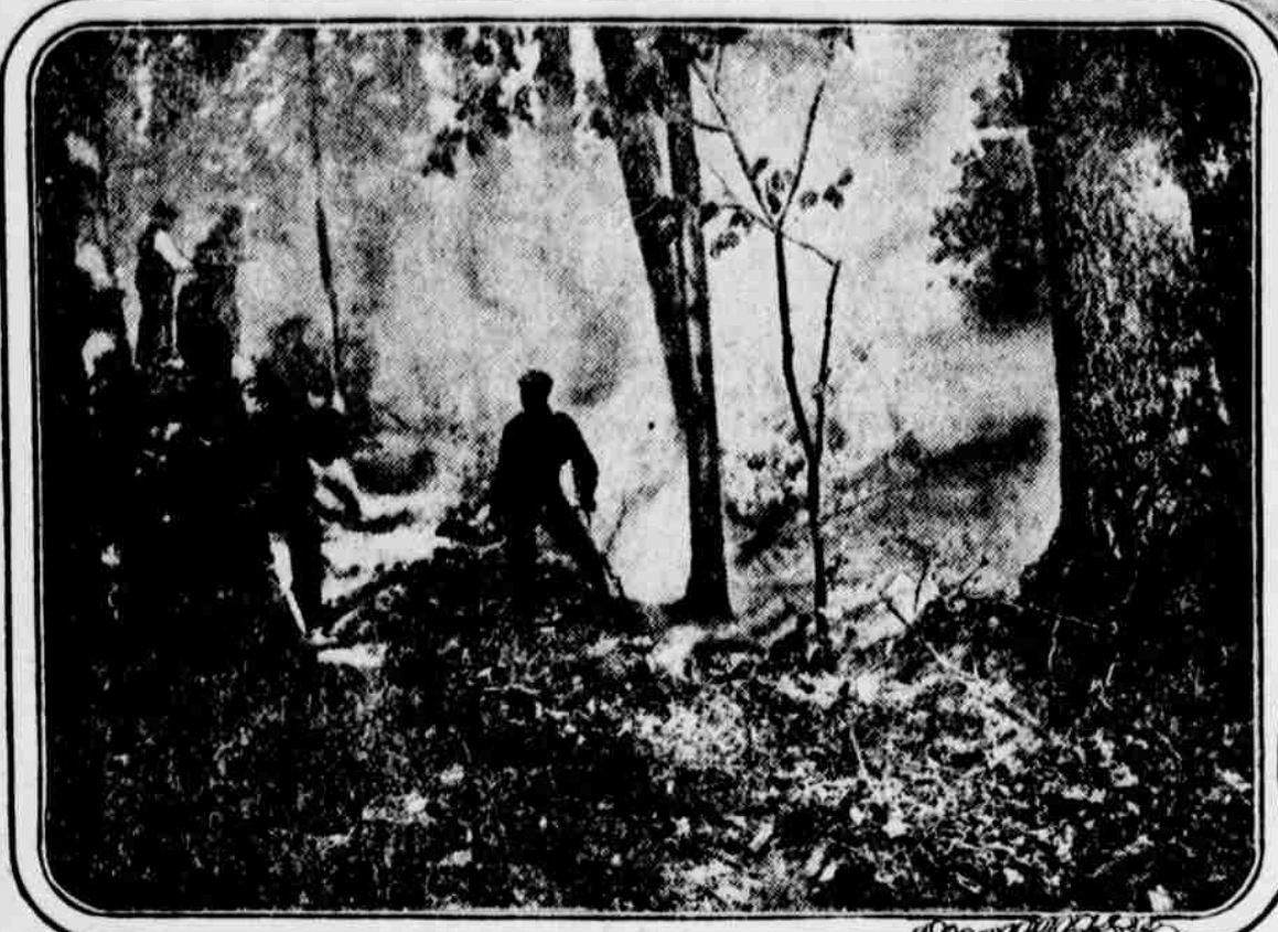
MAKING A TRENCH FROM WHICH TO FIGHT FOREST FIRE
