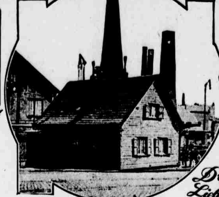
THE ORIGINAL KRUPP FACTORY
