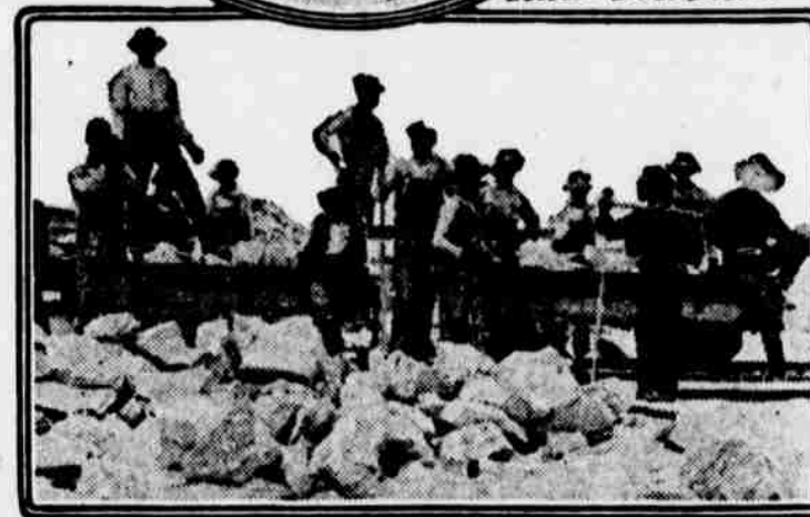
BEAKING STONE FOR A NEW ROAD
