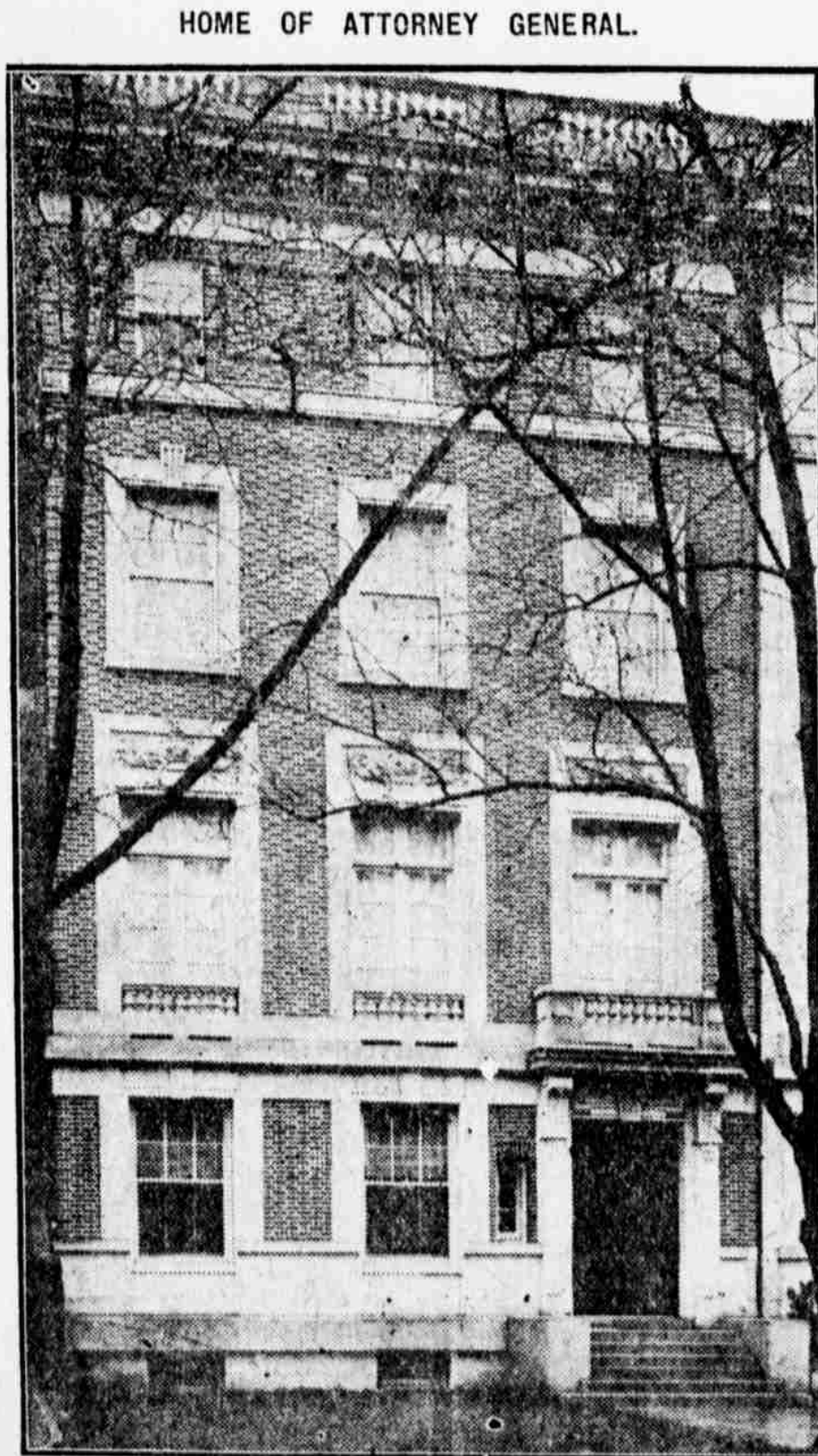
Residence of George W. Wickersham, Attorney General of the United States, at Washington.
