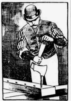
this device, asserts that an ax lends itself admirably for use as a brace as the heavy head forms a convenient grip for the hand and its weight makes it easier to operate.
