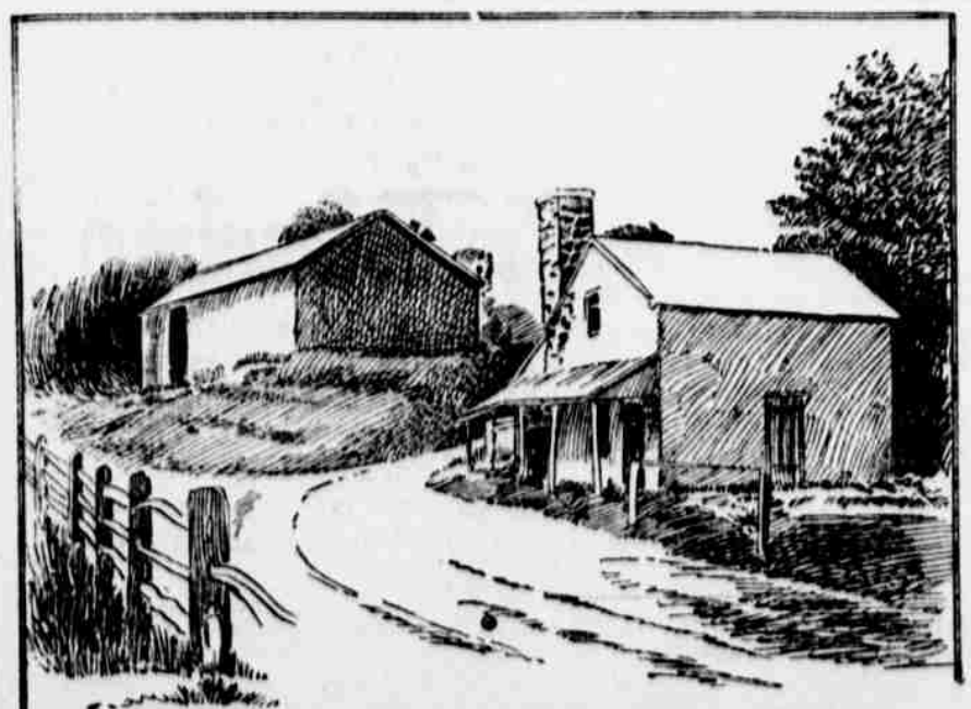
CHARCOAL HOUSE AND WORKMAN'S COTTAGE.
