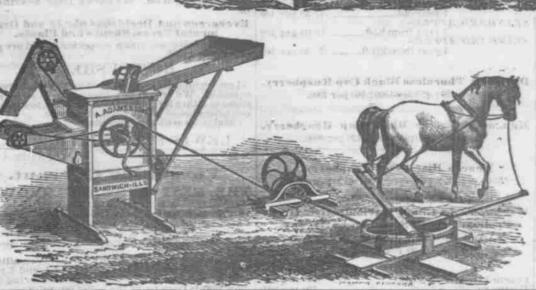
Two Hole Hand Feed Sheller (or "Farmer's Sheller") with one-horse power, jack and rope.
