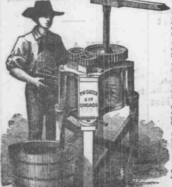
resseing 30 to 50 galions juice per hour. burse, weighs 650 pounds, and capable of ex-No. 2 is an upright three-roller mill, for per hour. Price \$65. No. 4 is an upright three-roller mill for gave a synopsis, two or four barses; weighs 1,400 pounds, and
