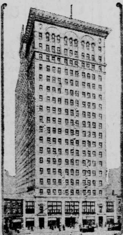
This is the big Y. M. C. A. hotel that has just been dedicated in Chicago, the first of its kind in the country. It cost $1,500,000, the money being donated by the business men of Chicago.
