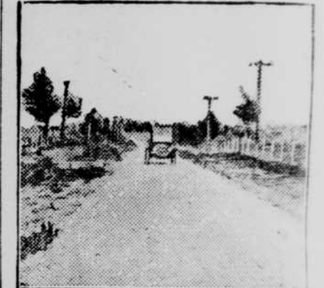
Well-Drained Road in Illinois.
