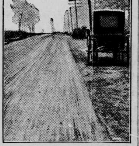
Road After Improvement With Top Soil Gravel.
