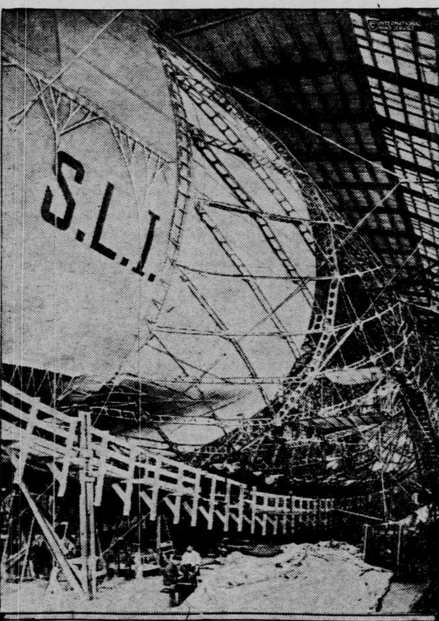
Scene in one of Count Zeppelin's workshops, where a giant dirigible is being constructed.
