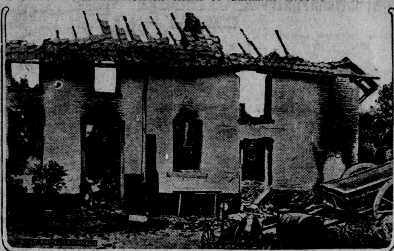
Blackened ruins of a burned farm house near Liege, destroyed by the German troops. This was but one of thousands of dwellings thus wrecked by the kaiser's soldiers.
