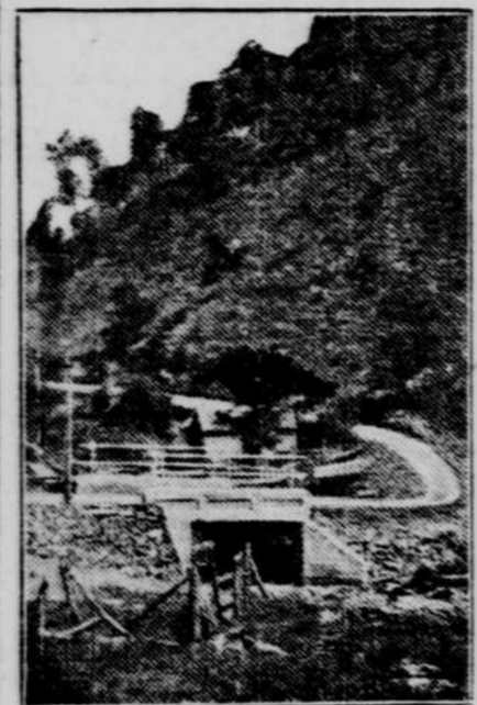
Concrete Culvert in Virginia on a Stretch of Macadam Road.
