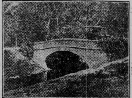
Concrete Arch Bridge in the District of Columbia.
