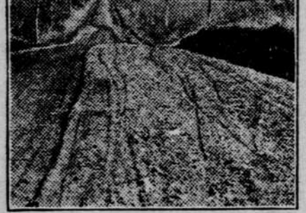
A "Chats" Road in Jasper County, Mo. "Chats" is a Term for Mill Tailings from the Mining District.
