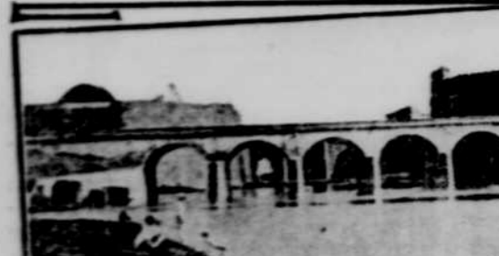
THE PIER OF SEAPORT AND BRIDGE AT DELHI.
