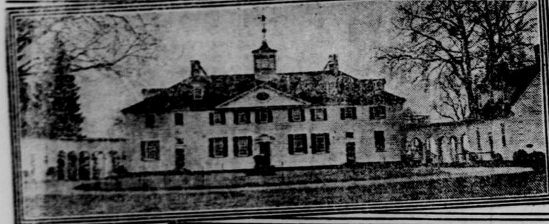
REAR OF MOUNT VERNON MANSION SHOWING THE NEW ROOF, COLONNADES, ETC.
