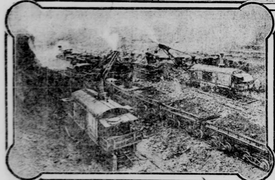
HALLING OFF EXCAVATIONS FROM CULEBRA CUT
