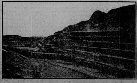
The above workings in the open air at Hongay, Tonkin, are on the side of a hul, which is one solid block of coal about 200 feet high. To get at the min-eral, it is only necessary to remove a layer of schist on the surface. The coal which is of a good quality, is mined to the extent of about 1,000 tons a day.
