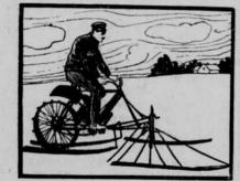
proper is about six inches, on the outer edge of which are broad teeth that are to give'the power in the snow or soft ice. In the center is a penumatic tire of rubber two inches wide. This is covered with steel wire to prevent puncture, and this latter is covered with a strip of leather which is filled with sharp steel teeth about the size of the head of an ordinary screw, that will grip the hardest ice and, as Mr. Wells put it, will climb the side of a house.
