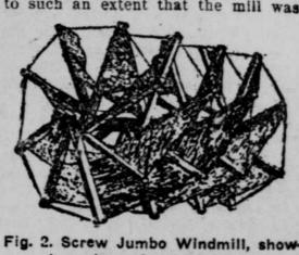
ing plan of construction. disqualified for use. Fig. 2 shows the construction of the mill. The sails of canvas are attached to arms of wood which are braced and tied together with twisted wire.
