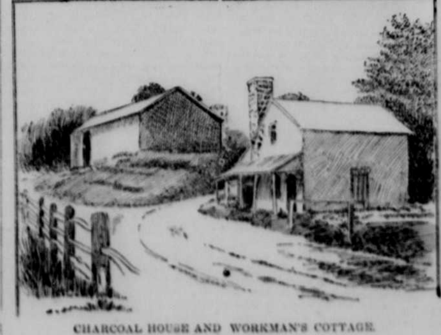
CHARCOAL HOUSE AND WORKMAN'S COTTAGE.
