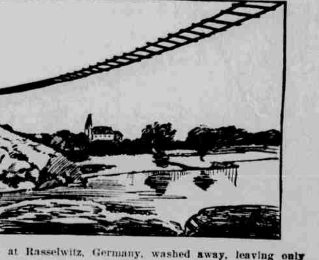
Railway bridge at Rasselwitz, Germany, washed away, leaving only rails and ties.
