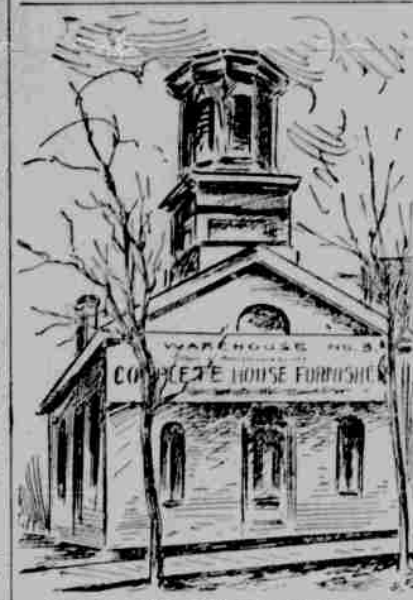
OLD CHURCH, NOW A WAREHOUSE.
