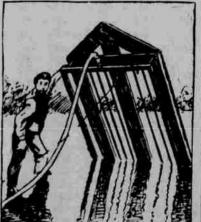
FLOAT FOR DISTRIBUTING OIL. destroys the floating larvae of the mosquito. During the process of distribution the float is pulled backwards and forwards over the ponds so that every inch of the surface is treated with petroleum. The ground around the pond has been cleared of rank vegetation, and the bank: have also been saturated with oil. Doctor Doty will now watch the health reports of his district for some indication that his experiment has been successful.-Pennsylvania Grit.
