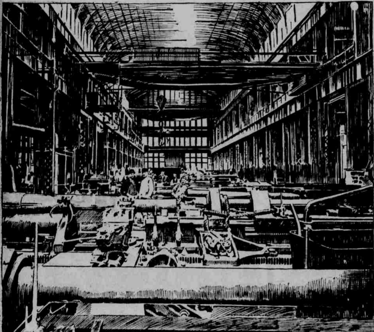
VIEW OF THE INTERIOR OF THE PRINCIPAL STRUCTURE.
