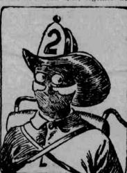
RESPIRATOR FOR FIREMEN. means for supplying air thereto, and mechanism by which the air can be brought from a distant point. A knapsack is attached to the back by straps, and connection is made with an alr tube paralleling the line of hose, the sir pump being located on the hose cart outside the building. If the line should become fouled the fireman can immediately stop any waste, and there will still remain a sufficient quantity
